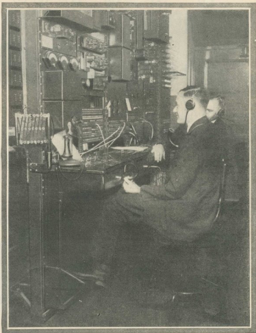
The operators at the New York switchboard during the transatlantic radiotelephone tests are here shown. © International Newsreel.
