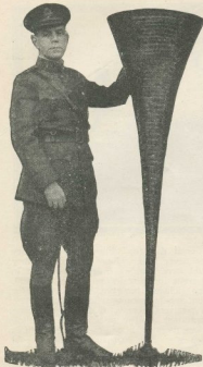
The author with a 6-foot exponential horn used for an experimental radio loud speaker.
