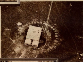
THE LEAD-IN TRUNK ON TOP OF THE STATION. The ring surrounding the trunk is the terminal of the ground plates. This system of counterpoise is considered one of the best known.
