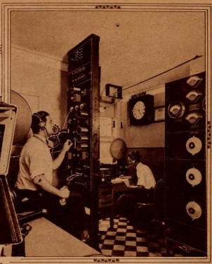
BATTERY-CHARGING PANEL. This panel, which was built by the station's staff of engineers, controls the charging of any or all of the storage batteries used in transmitting.
